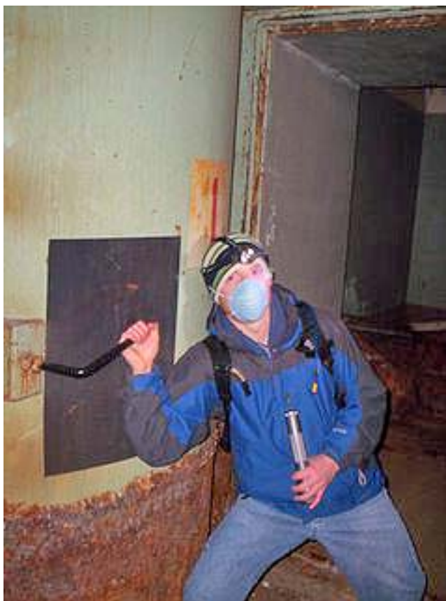
The first blast door between entrapment area and stairwell.
